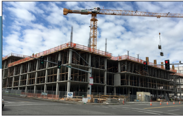
Photo courtesy of Sellen Construction Co.
