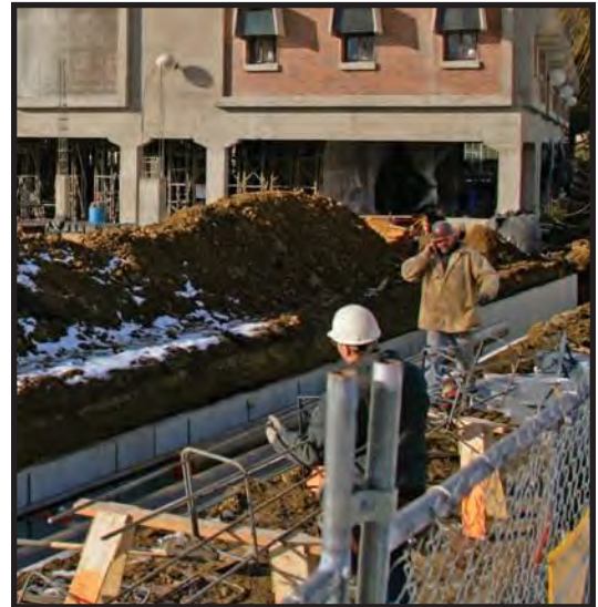
Work on “utilidors” near Dean Hall.
