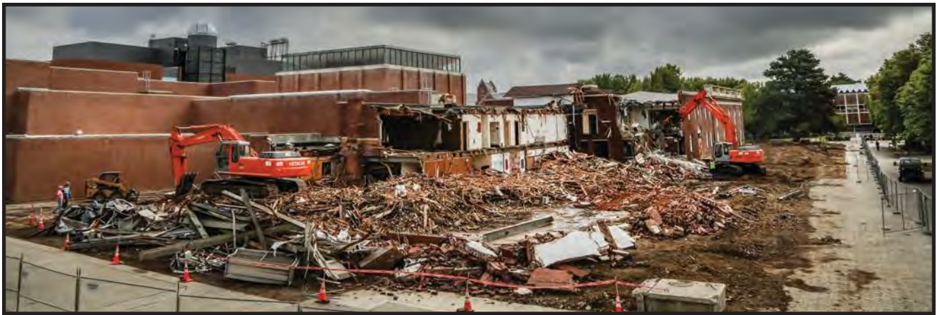
Remodeling and renovating Samuelson began with demolition of part of the original building.
