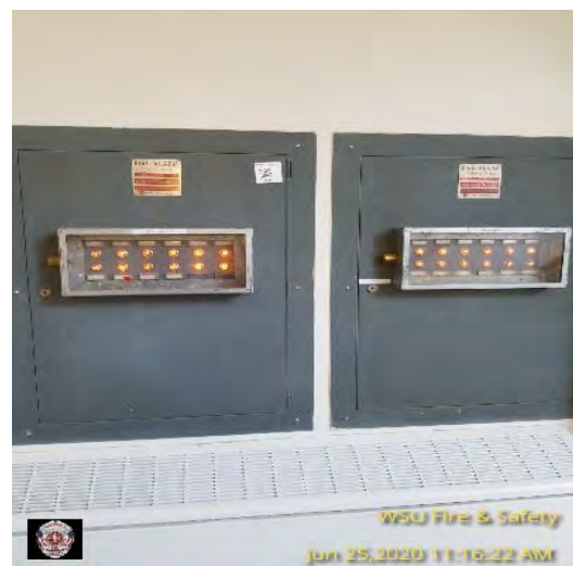
Figure 2 - Johnson Hall Fire Alarm Panel
