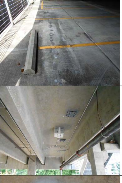
Photograph 7: Mineral deposits on the parking deck surface below the location in the previous image, from water dripping from the double Ts.
