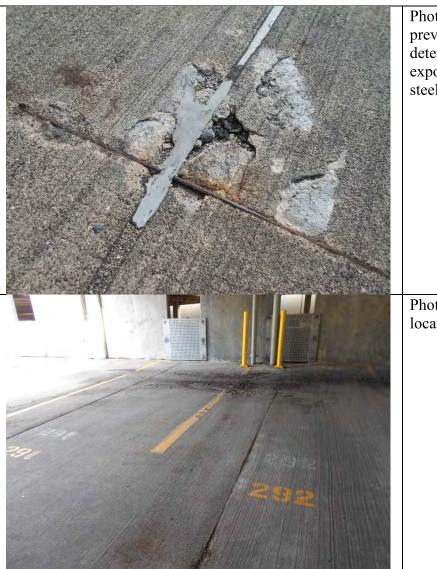
Photograph 25: Detail from previous image showing deterioration of joint edge and exposed and corroding reinforcing steel.
