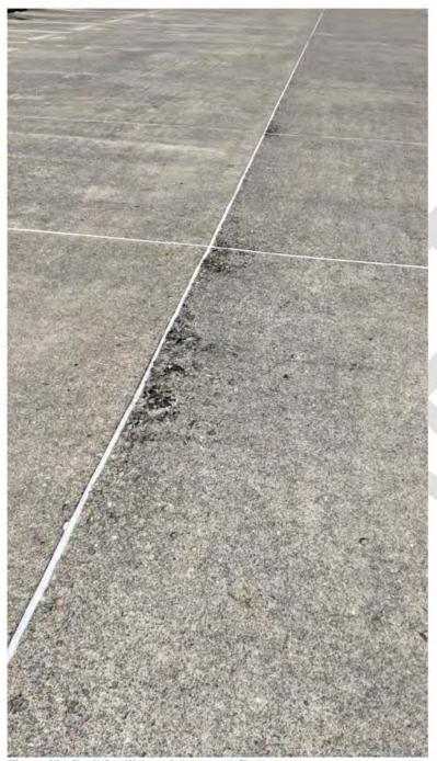
Figure 20 - Deck Spalling and Aggregate Exposure
