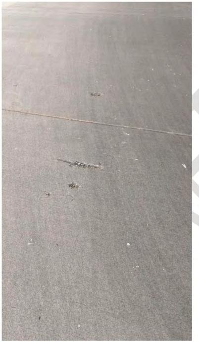
Figure 17 - Minor Spalls in Deck
