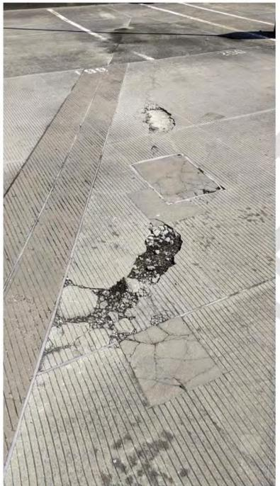
Figure 28 - Cracking, Spalling and Potholes in Upper Level Deck
