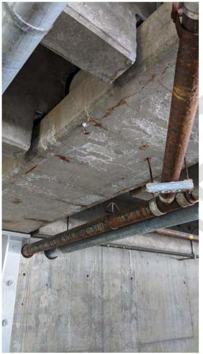
Figure 26 - Severe Cracking with Efflorescence and Rust Staining - Upper Level Girder
