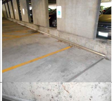
Photograph 10: Sheet metal flashing installed at the interior termination of the topping slab, level 1.
