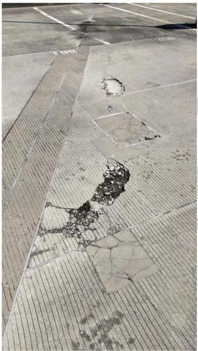
Figure 29 - Cracking, Spalling and Potholes in Upper Level Deck
