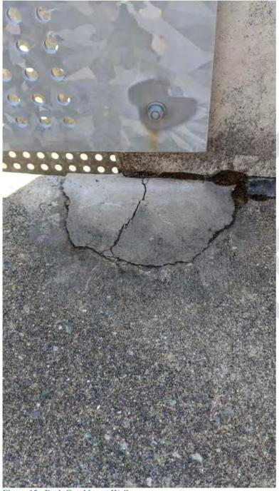
Figure 15 - Deck Cracking at Walls
