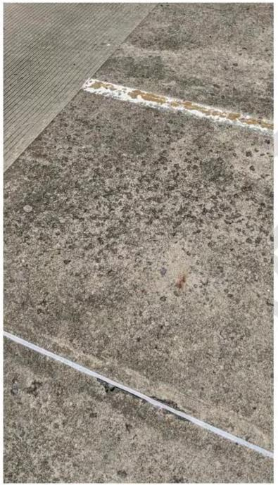
Figure 21 - Deck Aggregate Exposure
