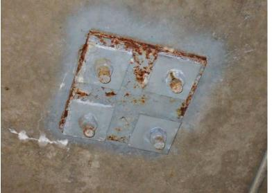
Photograph 9: Detail view from previous image, showing corrosion of the plate. This condition should be addressed at the time of repairs.
