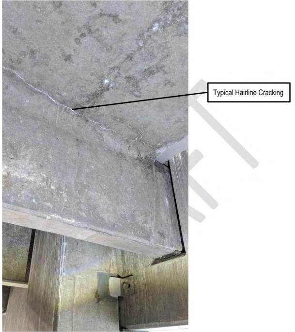
Figure 6 - Typical Hairline Cracking in Double-Tee Beams
