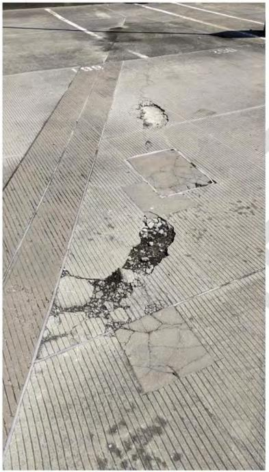
Figure 24 - Cracking, Spalling and Potholes in Upper Level Deck
