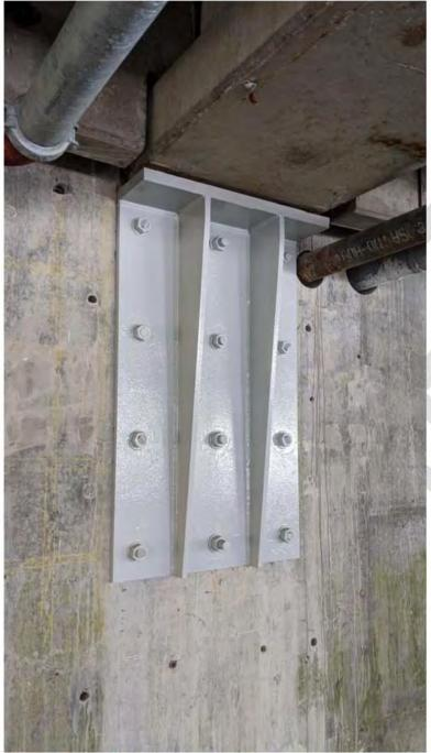
Figure 25 - New North Corbel Supporting Upper Level Girder
