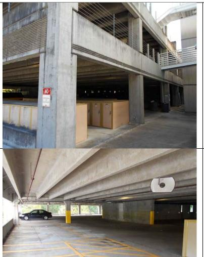
Photograph 4: West elevation overview, showing precast columns and beams.
