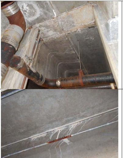
Photograph 28: Efflorescence and corrosion of steel elements resulting from inward migration of water through concrete structure elements.
