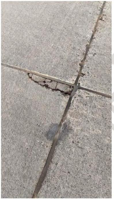
Figure 13 - Deck Crack at Intermediate Joint
