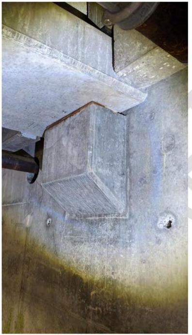
Figure 5 - First Floor Corbel - South End of Garage
