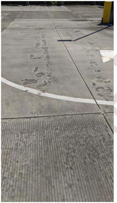
Figure 23 - Water Stained Low Spots in Overlay
