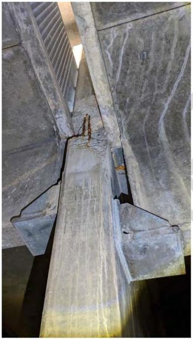
Figure 9 - Center Wall Spall (appears to have been patched and re-spalled)
