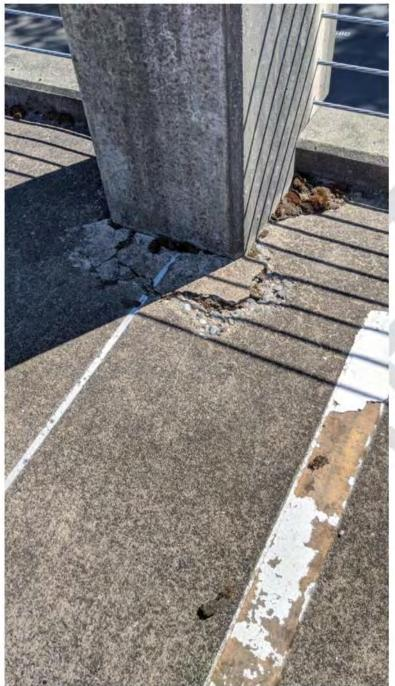
Figure 14 - Deck Cracking at Columns
