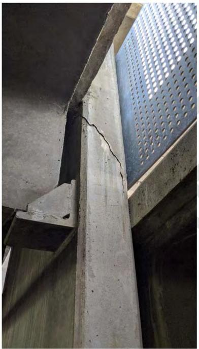
Figure 11 - Center Wall Diagonal Crack
