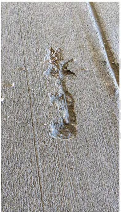
Figure 18 - Minor Deck Spall with Exposed Reinforcing
