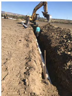
Conversion of 960 acres from rill to sprinkler irrigation (above) including the installation of nearly 40,000 feet of pipelines to date.
