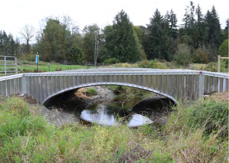
Removing fish barriers and replacing them with bridges that allow fish access.
