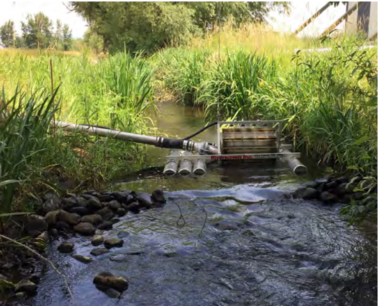
Installing fish-friendly screens on irrigation intakes.
