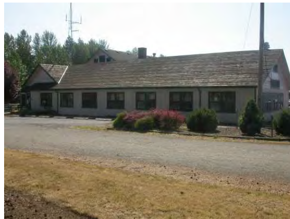
secondary structure, another view
