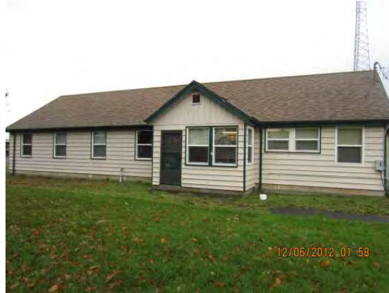
J:\facilities\Projects\PC Region\PC0602 Chehalis Survey Building - Roof\1392.JPG
