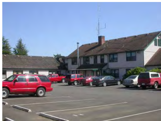
secondary structure on site, another view
