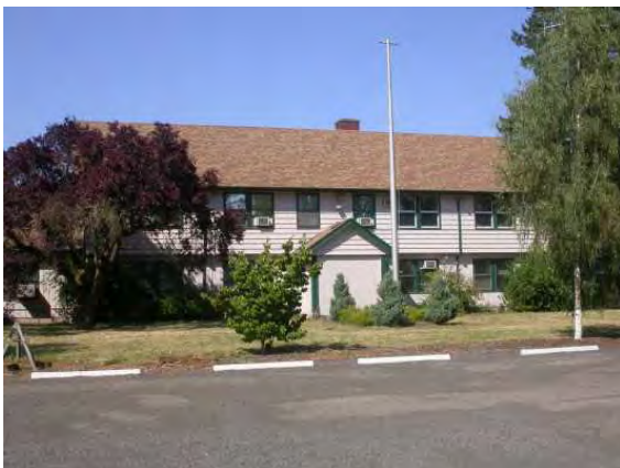
secondary structure on site, another elevation of structure
