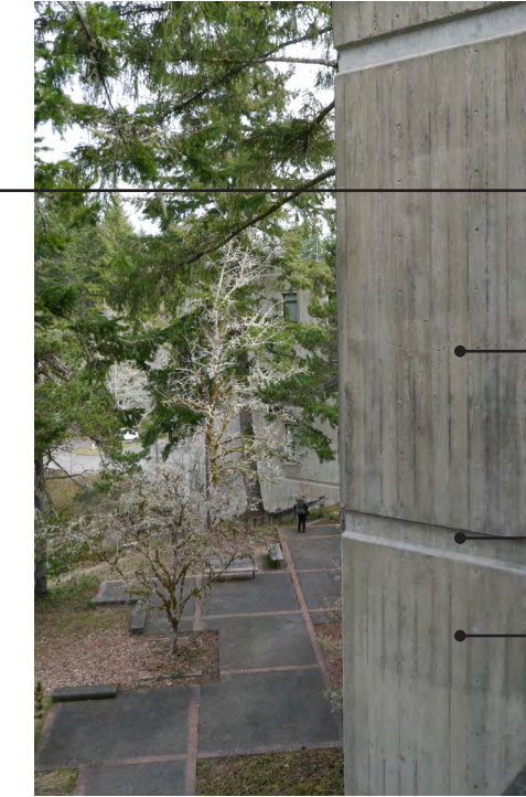
TYPICAL EXTERIOR WALL
