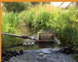
Installing fish-friendly screens on irrigation intakes.
