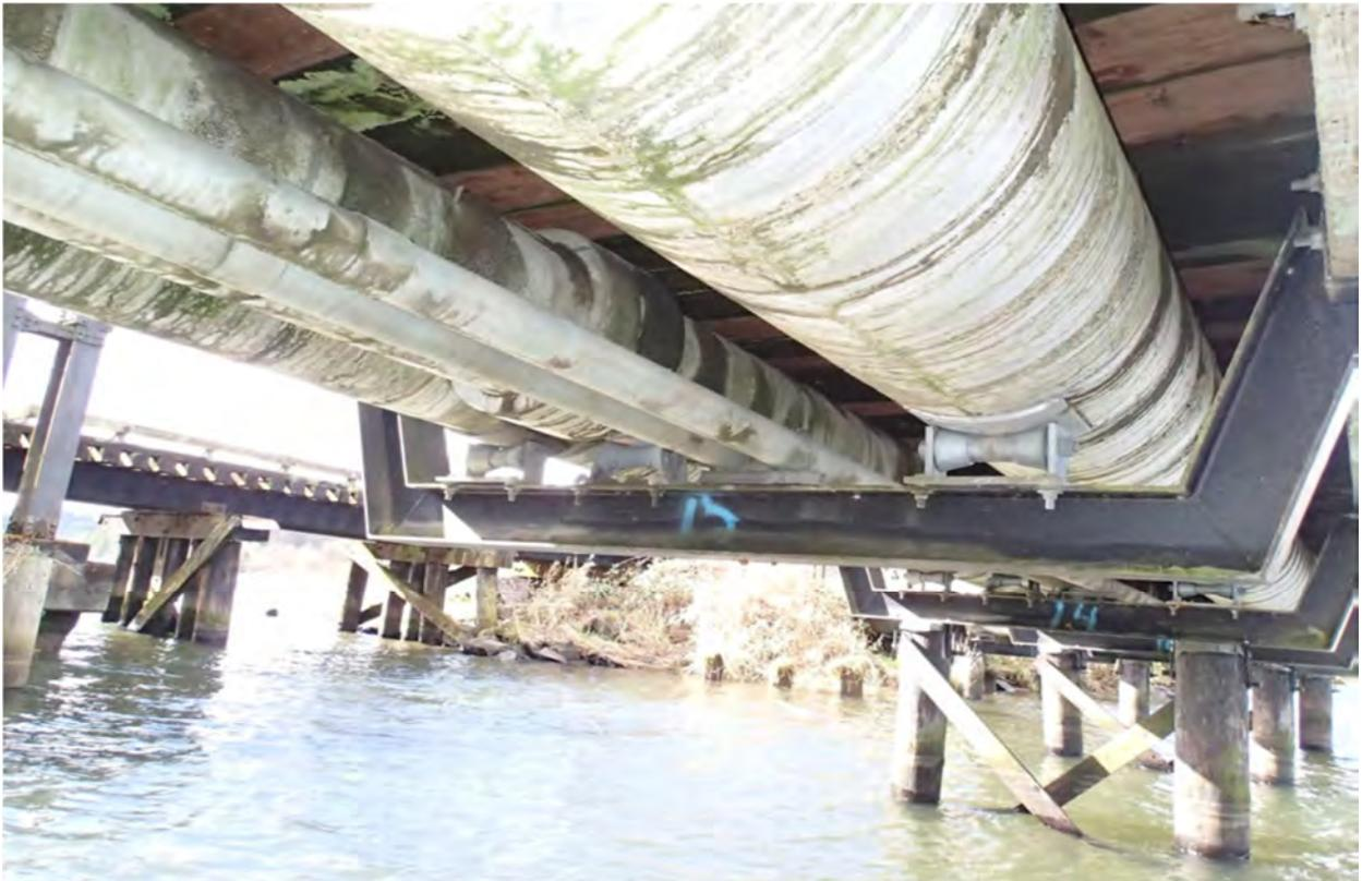
Photo 3 - Typical abandoned bolt holes in piling and section loss in bracing member
