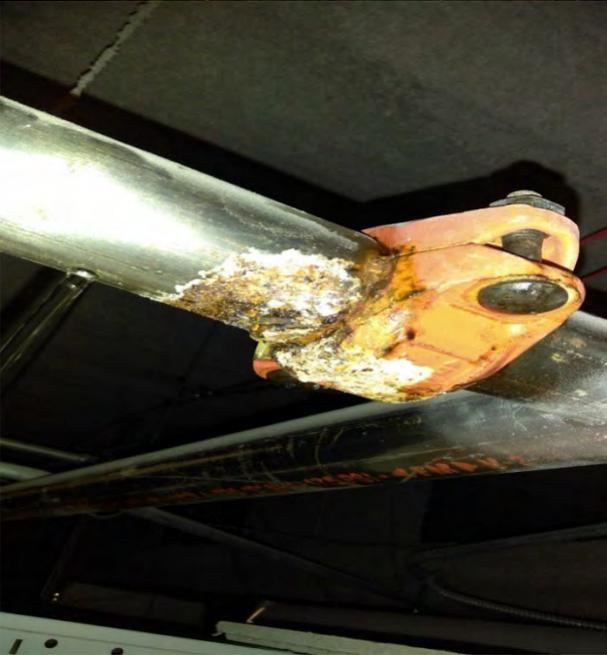
Exhibit C: Fire sprinkler piping actively leaking.
