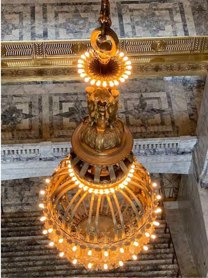
The chandelier, which weighs 10,000 lbs., and measures 8' in diameter, is suspended 25' above the Rotunda floor from a 101' chain reinforced with a Kevlar rope.
