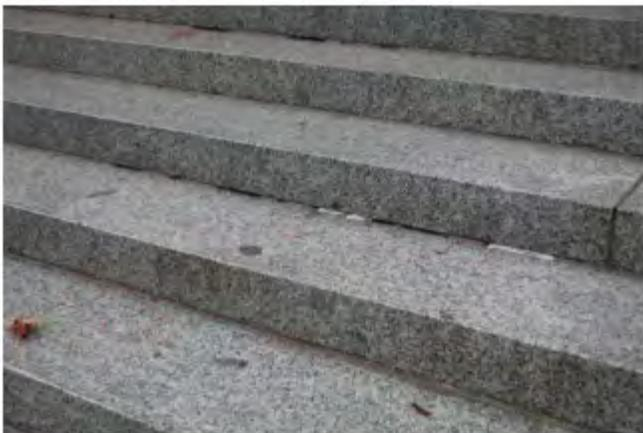
Figure 61. Granite steps with failing and missing mortar, and recent sealant repairs
