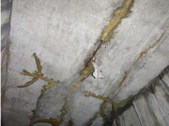
Exhibit C – Corrosion from water infiltration (2023)
