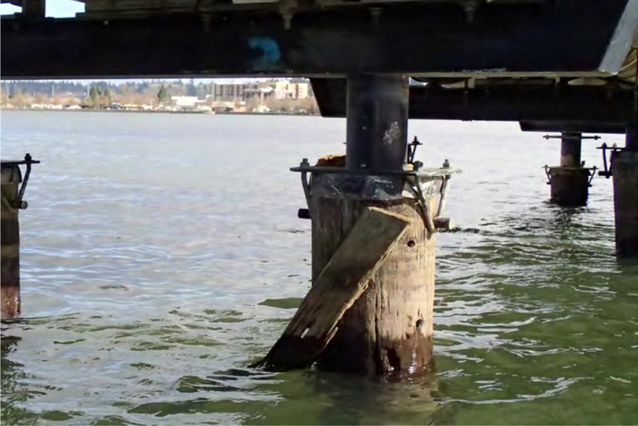
Photo 4 - Typical two-pile pier configuration
