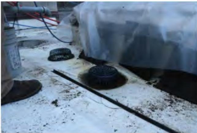
Figure 51. Roof drain and overflow above area of leak in the North Vestibule.
