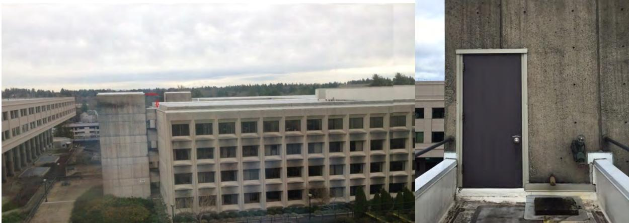
Covered ladders should be installed and single fall arrest anchor point centered on each of the four roofs.
