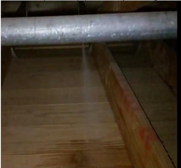
Exhibit B: Heavy corrosion at a sprinkler pipe connection.
