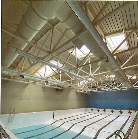
Stenehjem Fitness Center Pool Lighting
