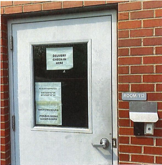
Ogden Resource Center Loading Dock
