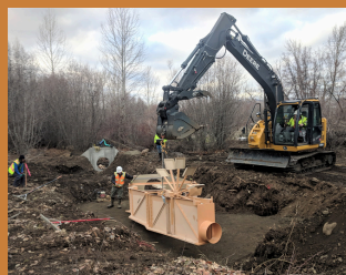
Installing fish-friendly screens on irrigation intakes.
