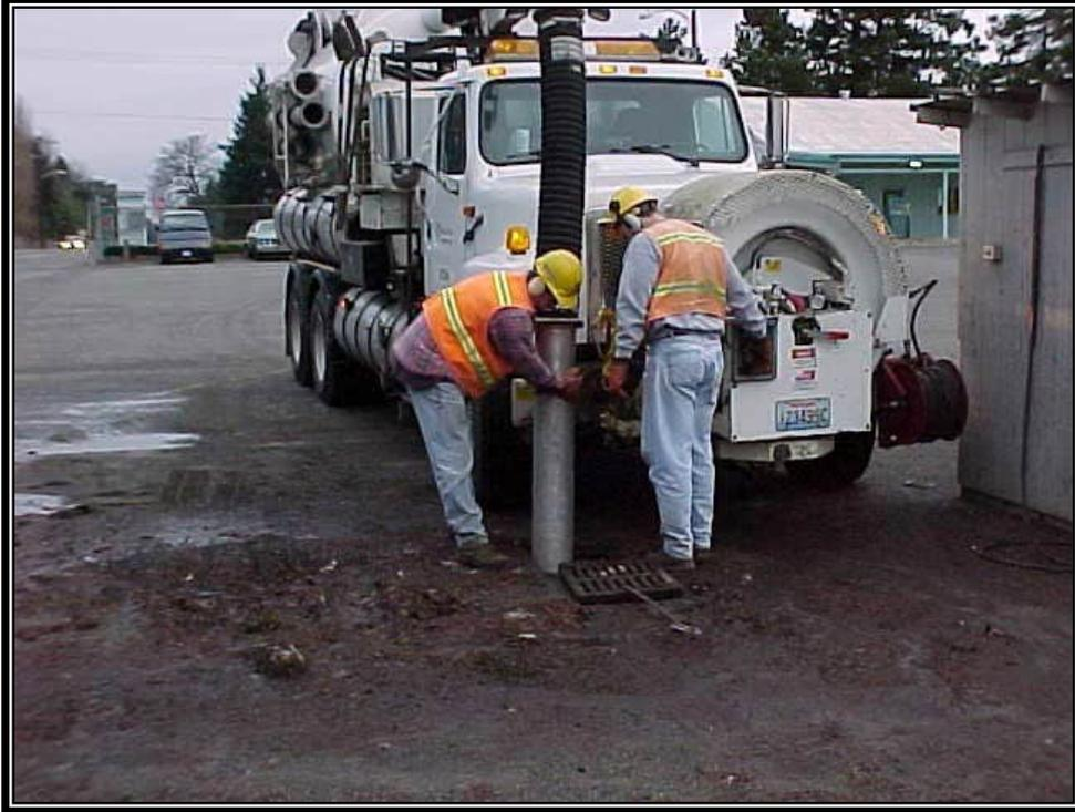
Figure IV - 4.23 Catch Basin Cleaning with a Vacuum Truck.
