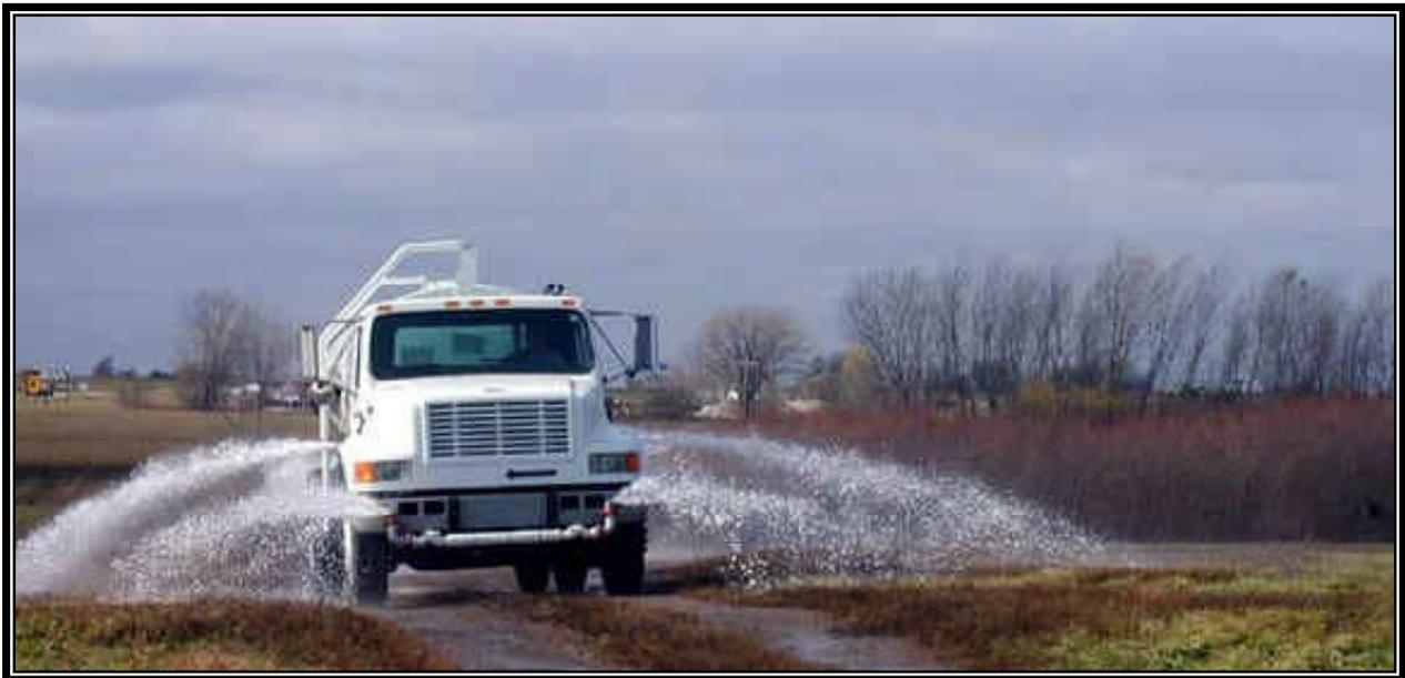
**Figure IV - 4.21 Dust Suppression by Water Spray.**
