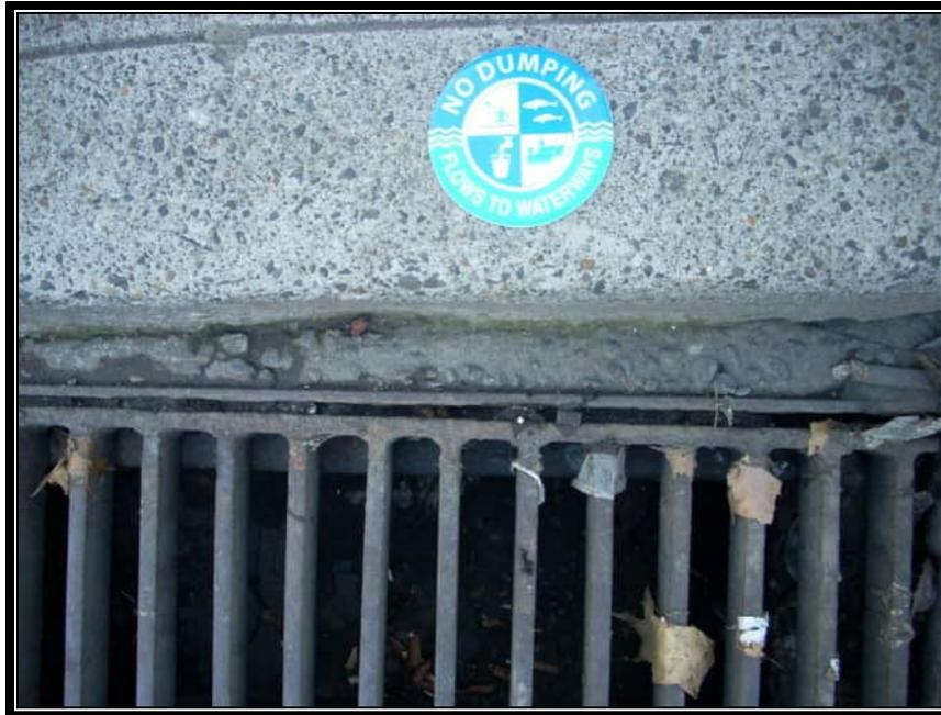
Figure IV - 4.24 “No Dumping” Storm Drain Button.
