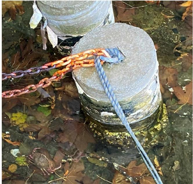
**Figure ES-2. Existing Concrete Anchors Used to Secure the Lagoon Dock.**
