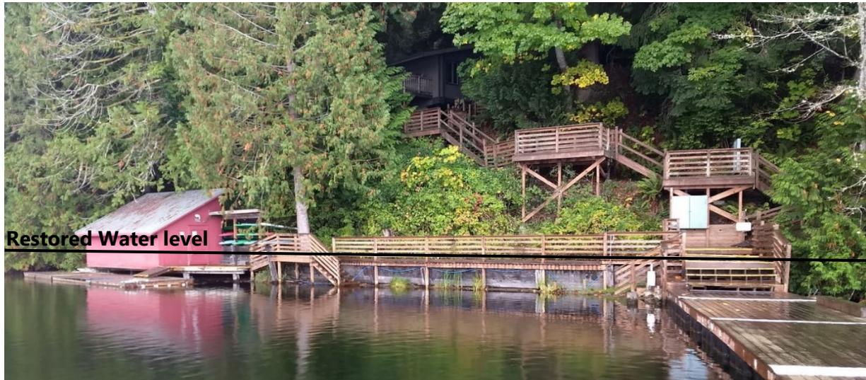
**Figure 5. Gangway, Decking, and Access Stairs Will Need to be Rebuilt to Accommodate Restored Water Level.**
