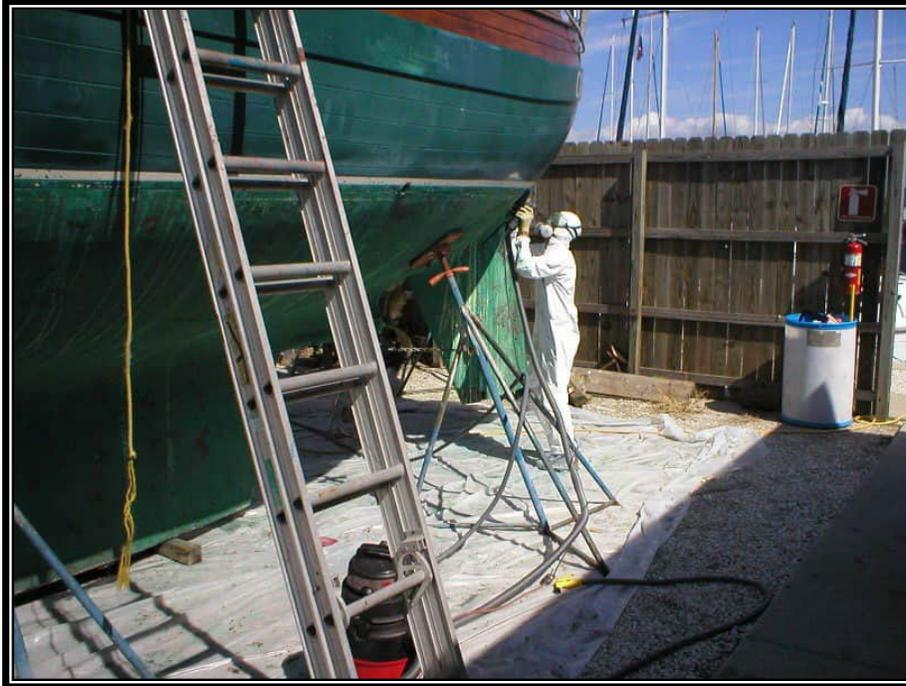
**Figure IV - 4.22 Drop Cloth Used During Hull Sanding.**
