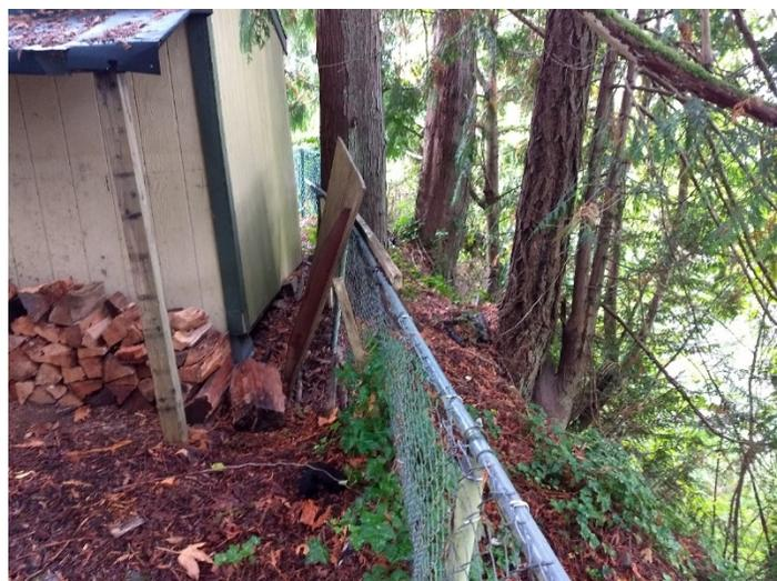
**Figure 8. Shed at the Firepit, Very Close to the Edge of an Undermined Bluff.**
