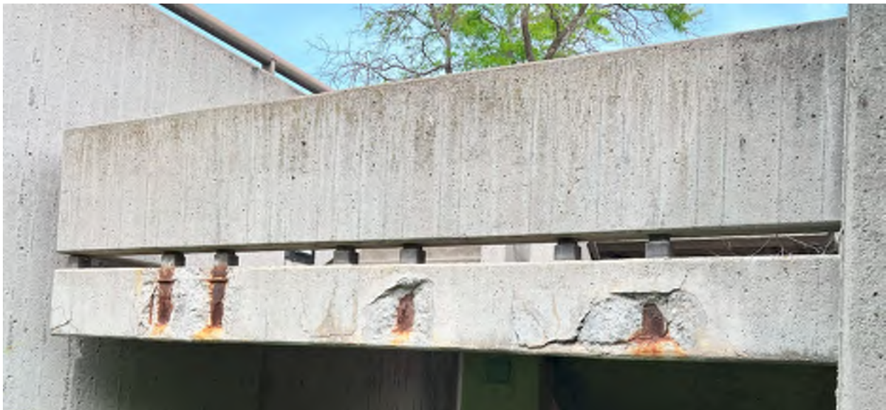
Spalling concrete at PEA Stair
