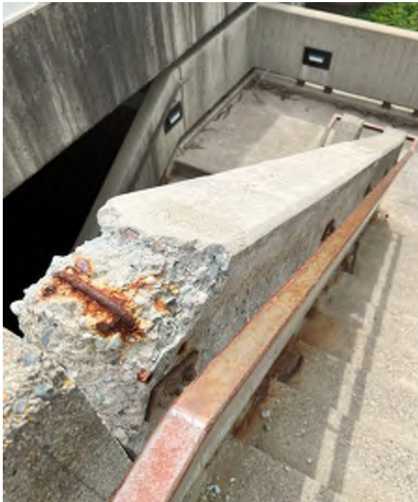
Deteriorating concrete at PEA Stair
