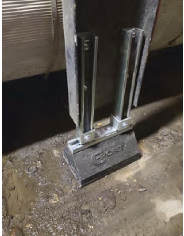
Proposed Support Stand Repair Actual Mock-up Installations
