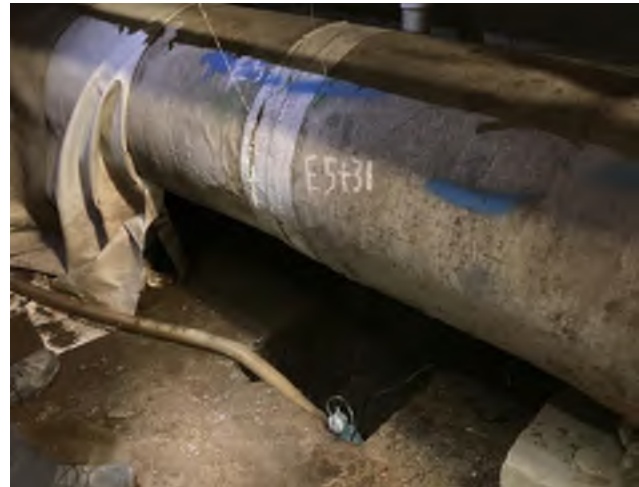
Fire hose discharge directly on to tunnel floor from nearby sump pump
