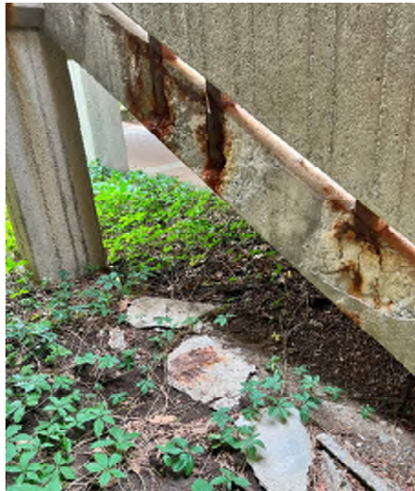
Spalling concrete at PEA Stair
