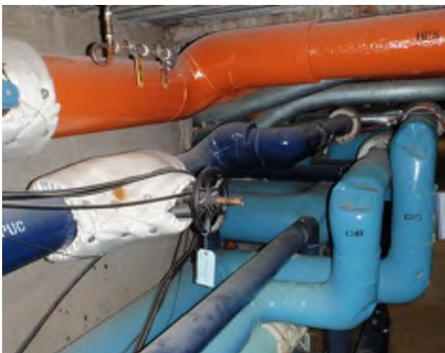
Example Existing Inconsistent Pipe ID Labels, Color Coating and Tunnel Address Marking on Pipe
