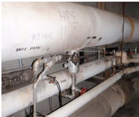
Example Existing Inconsistent Pipe ID Labels, Color Coating and Tunnel Address Marking on Pipe
