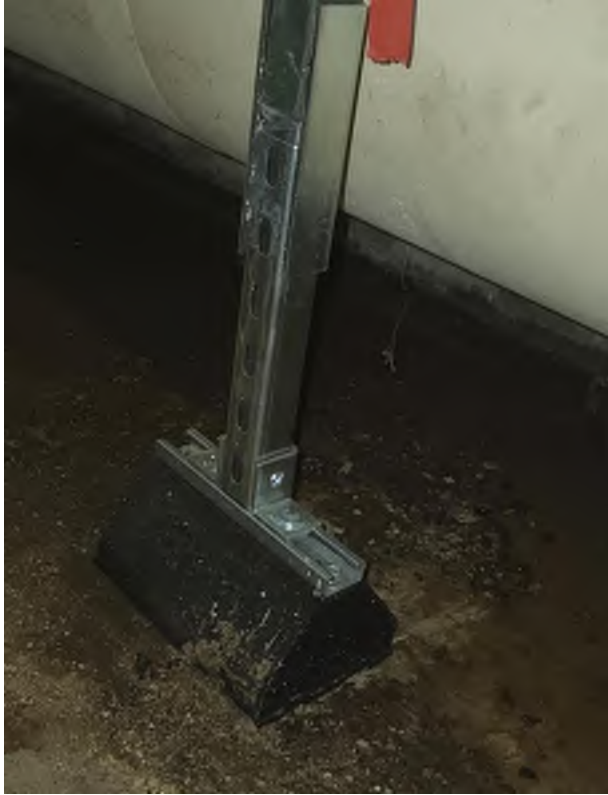
Proposed Support Stand Repair Actual Mock-up Installations
