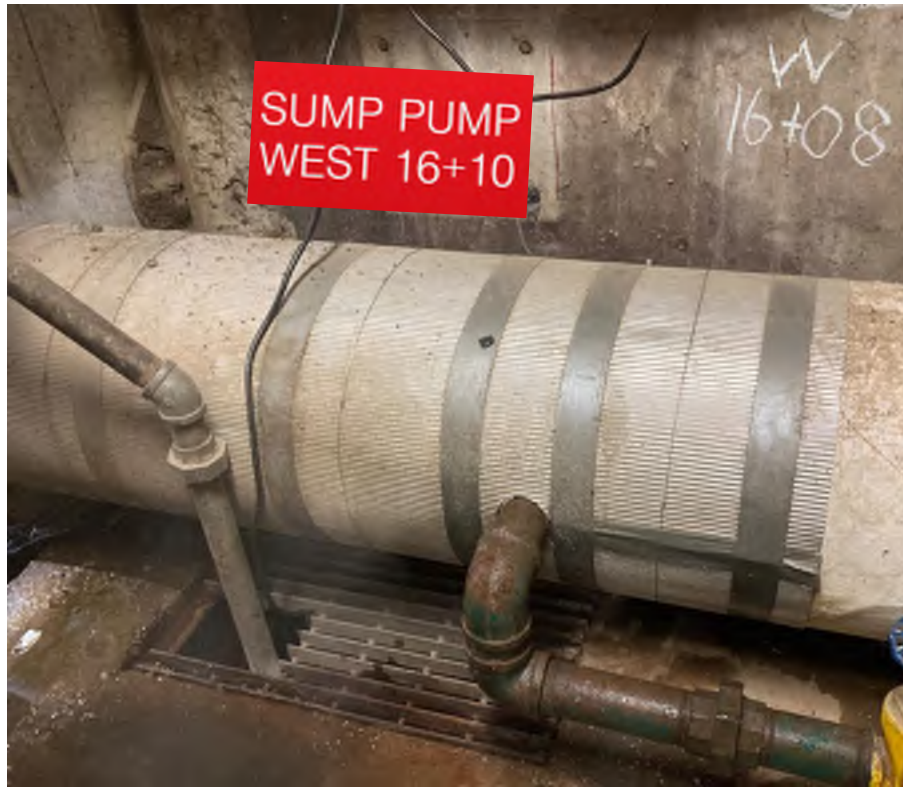
Example Tunnel Location “Road Sign” for Key Equipment Location
