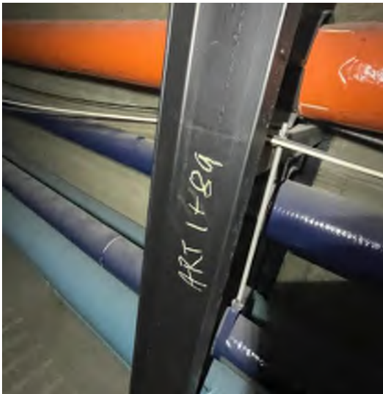
Example Field Survey Station Numbering “Chalk Marks” on Pipe Support Stanchions
