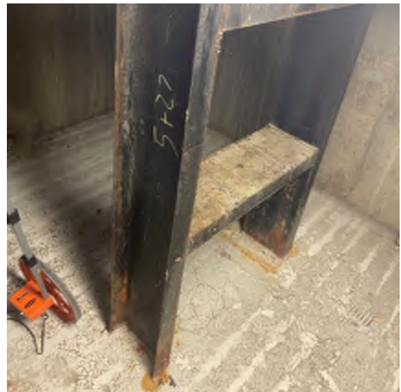
Example Field Survey Station Numbering “Chalk Marks” on Pipe Support Stanchions
