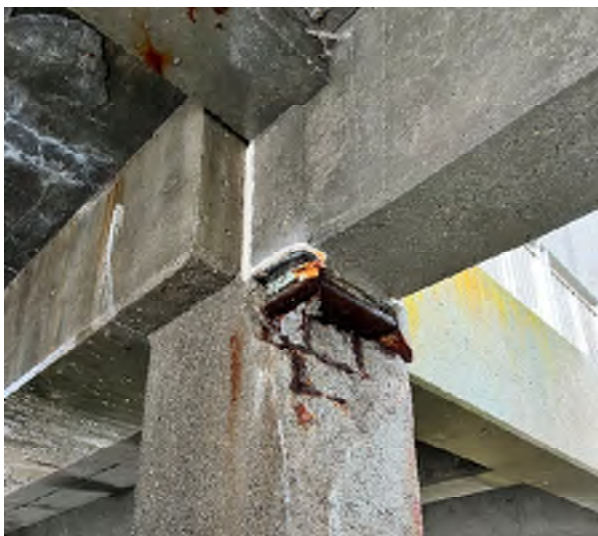
Damaged column at JFK ramp
