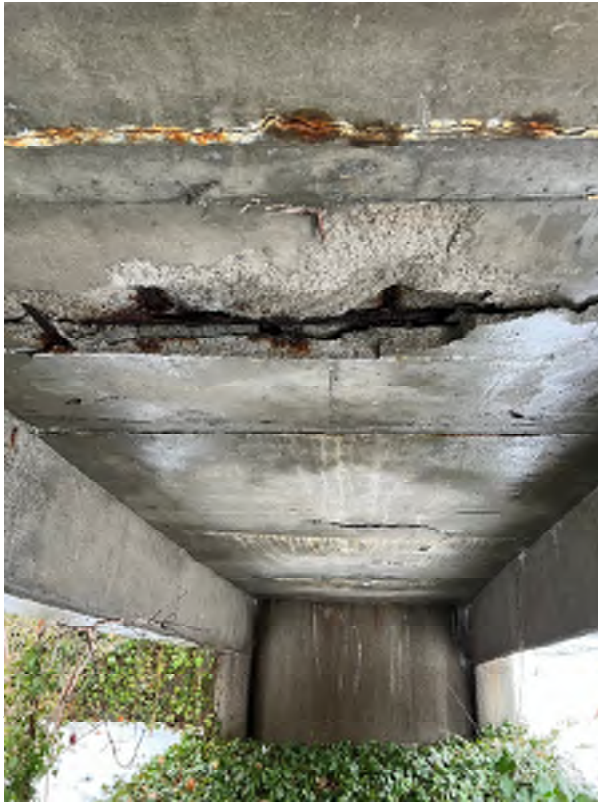
Spalling concrete, underside of JFK ramp
