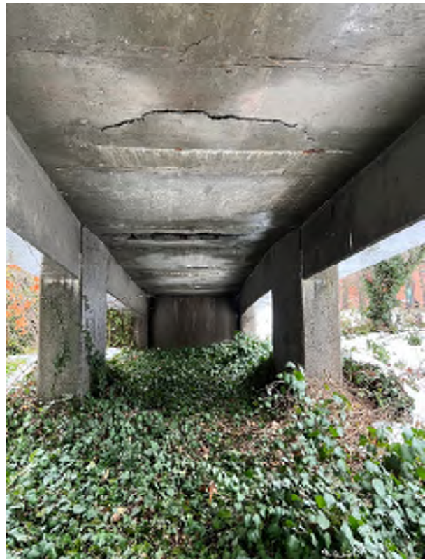
Spalling concrete, underside of JFK ramp
