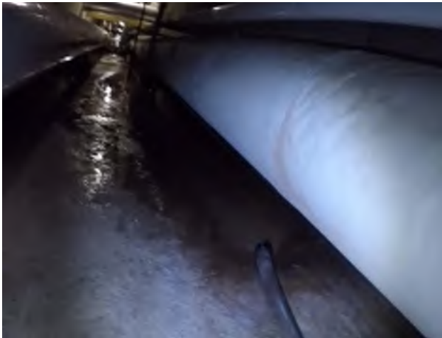
Fire hose discharge directly on to tunnel floor from nearby sump pump
