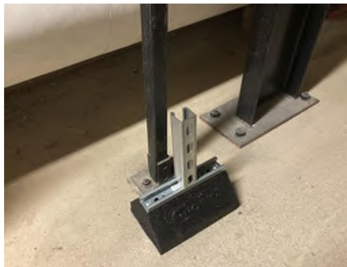
Proposed Pre-Fabricated “Roof Mounting Bases” for Stand Repairs
