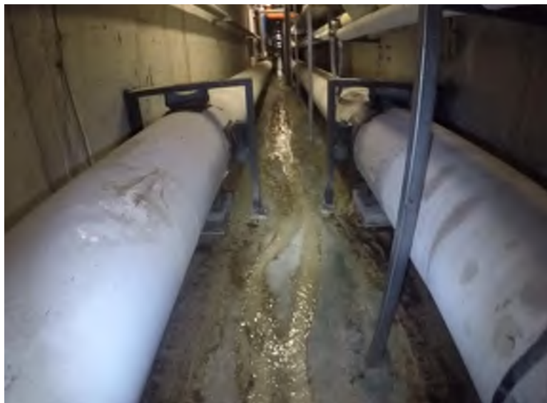
Problematic dewatering discharge stream running down tunnel floor
