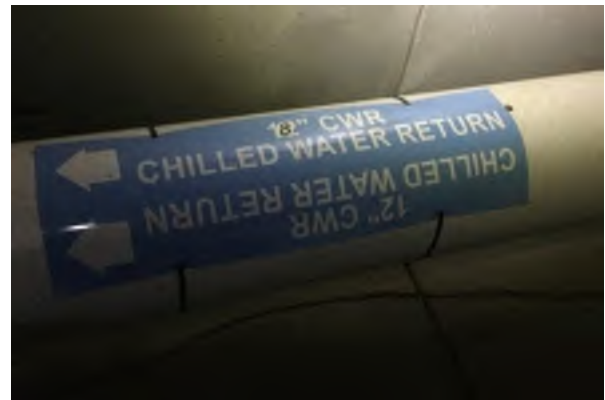
Example Tunnel Pipeline ID & Flow Direction Labels from ISC Tunnel Project
