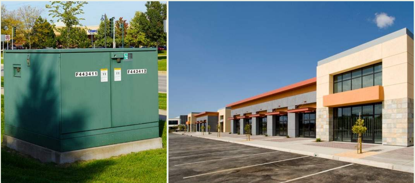
FIGURE 6. This large suburban shopping mall is served by seven units of pad-mounted gear in two looped-primary circuits. Two lineups of metal-enclosed switchgear are applied at primary-selective service-entrance switching centers to switch the ends of the loops.
