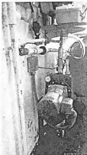
Upper pressure zone pressure pump
