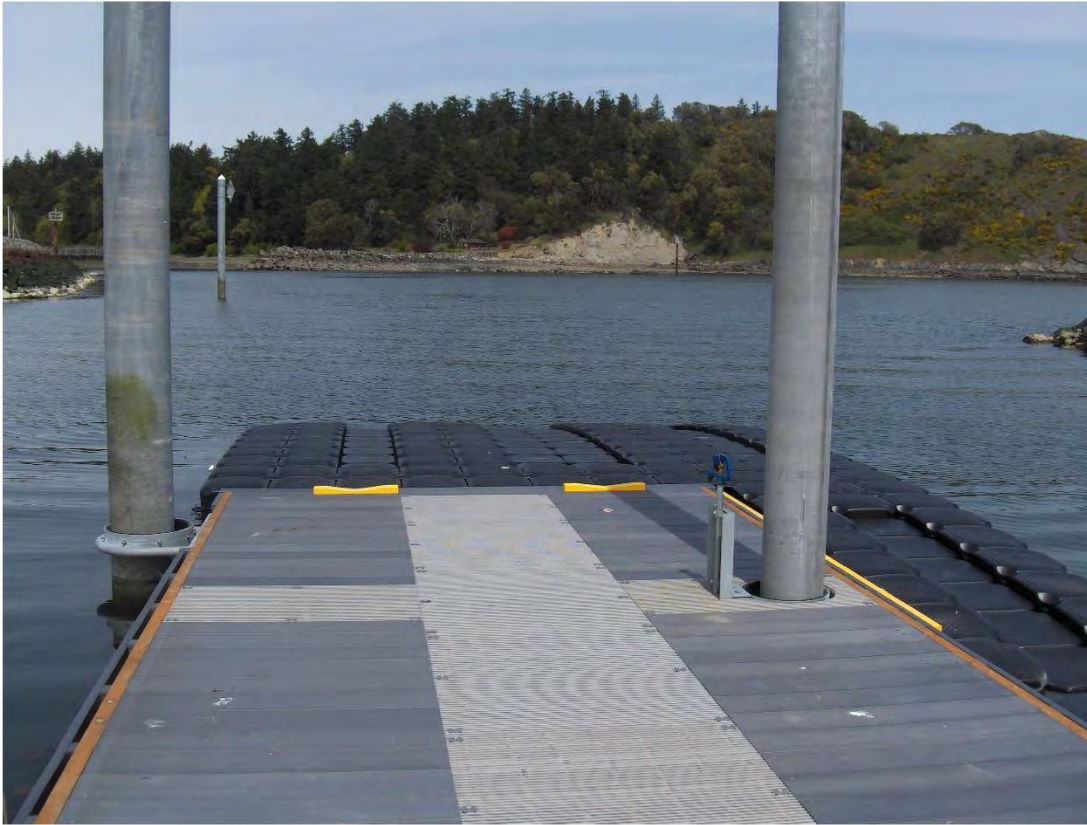
Figure 5. Hand carry launch system (Port of Anacortes Cap Sante)
