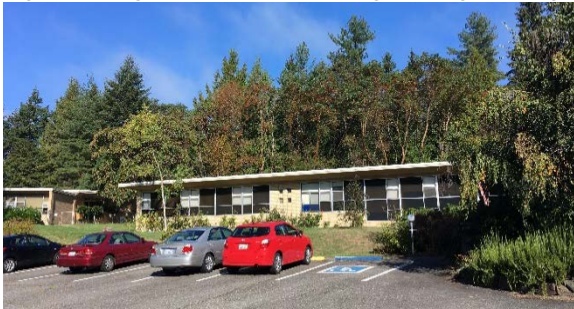
Figure 5 Image of one of the existing nursing buildings
