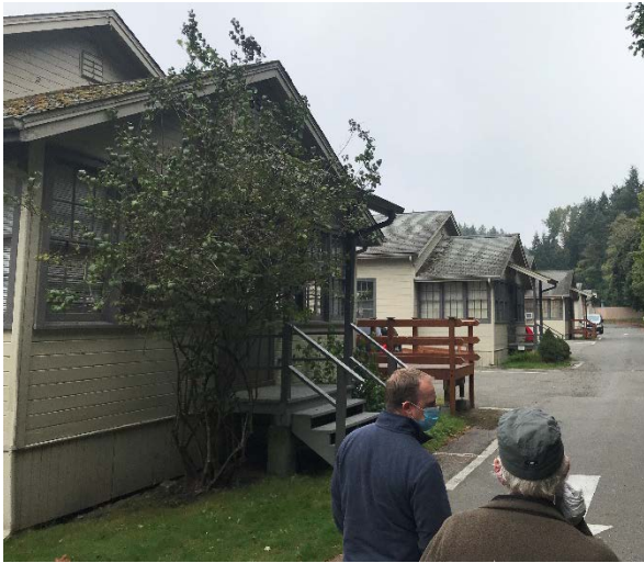
Figure 6 Image of the existing ATP building
